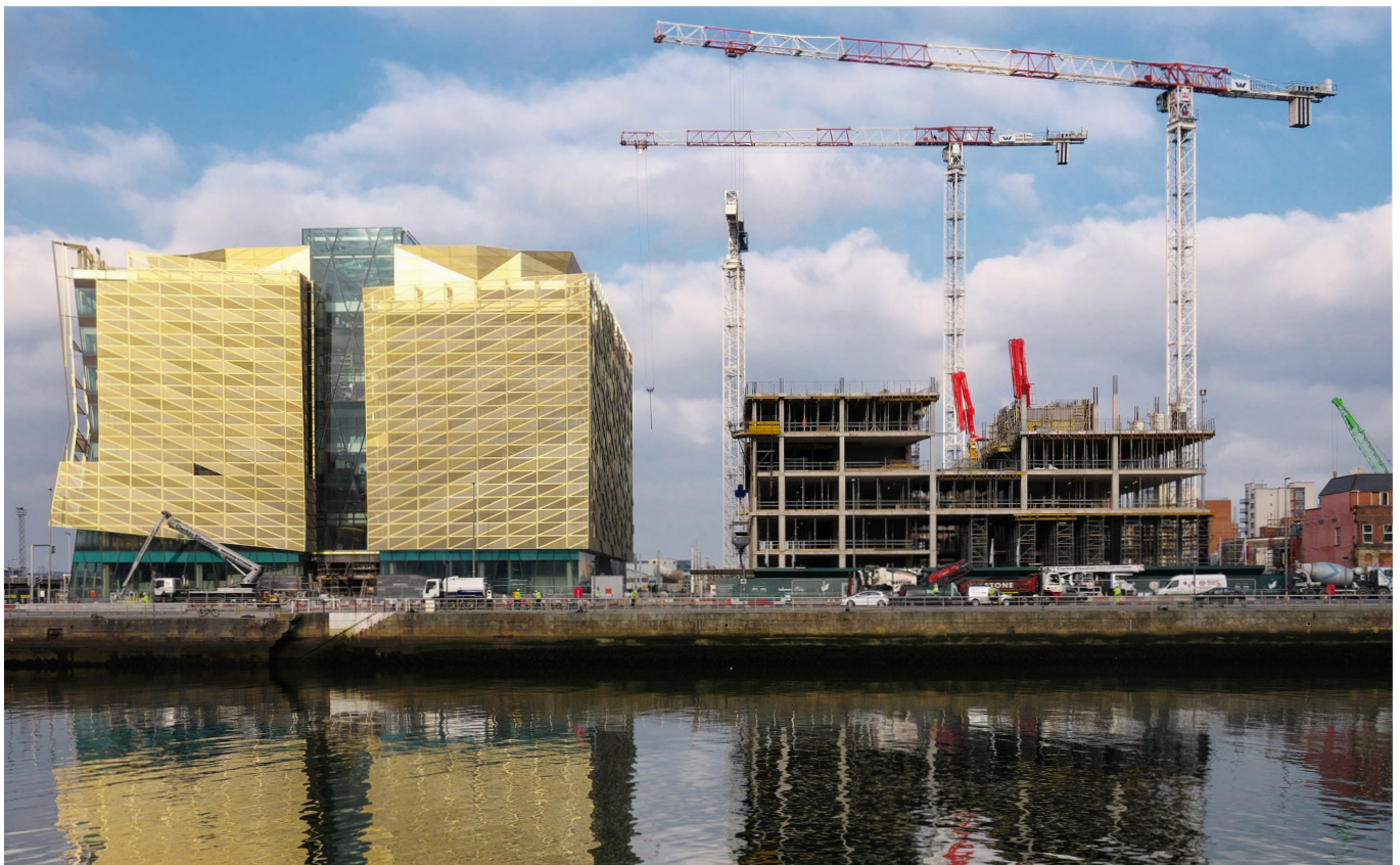
Constuction in the Dublin Docklands, January 2018
