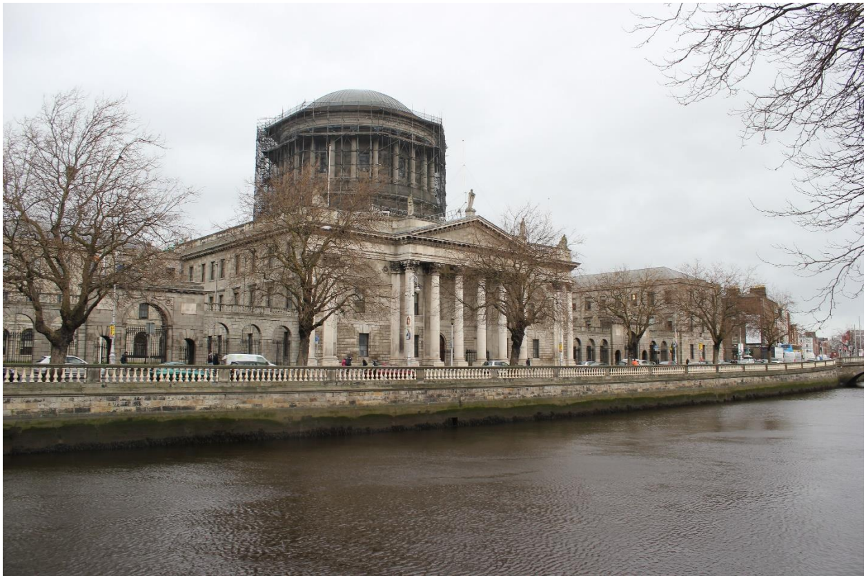
Photograph 5. Four Courts (photograph taken from opposite side of River Liffey).
