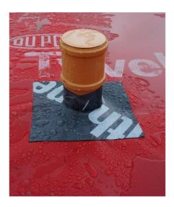
"Top hat" seal around services passing through the radon barrier
