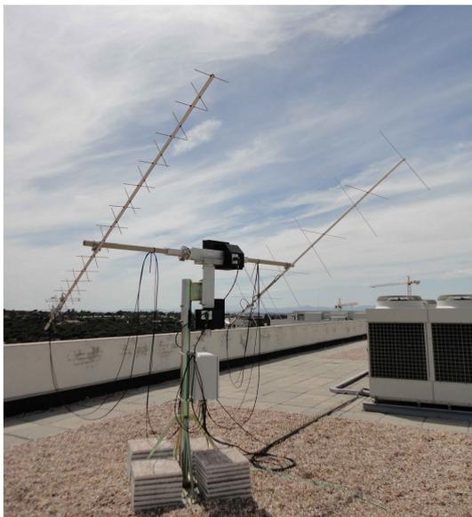
*A rotatable/tracking antenna for satellites*
